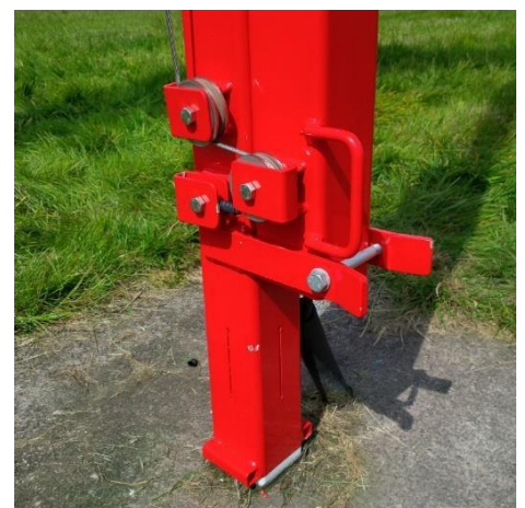
Securing Bolt & Winch Cable at base of mast
