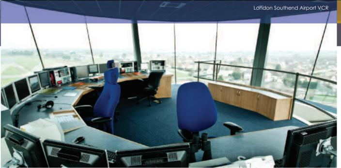
The variety of systems is evident in our projects, which typically involve the supply, installation and integration of fully fitted ATC Consoles, VHF/UHF Radio Communications and Airport Remote Monitoring Systems.
